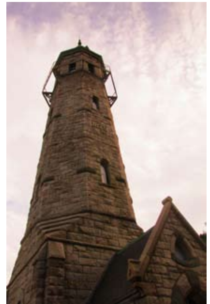
Fall River's old watertower near North Watuppa Pond
